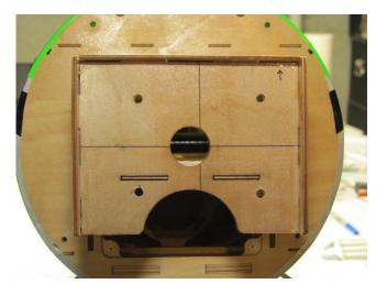
Remove template after drilling engine mounting holes.
